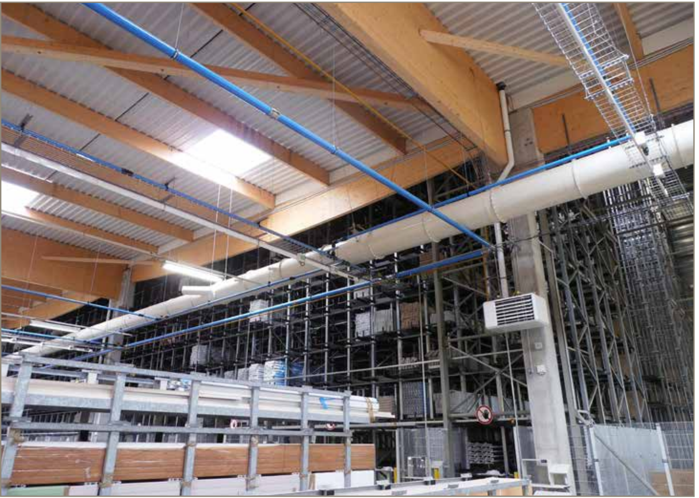
Transair® diameters from 25 mm (1") up to 100 mm (4")
